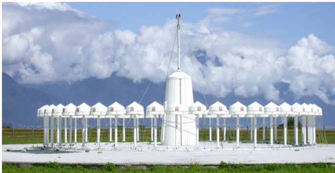
Figure-5.15 VOR-DME GND station left:[K4-6] right:[K5-1]
