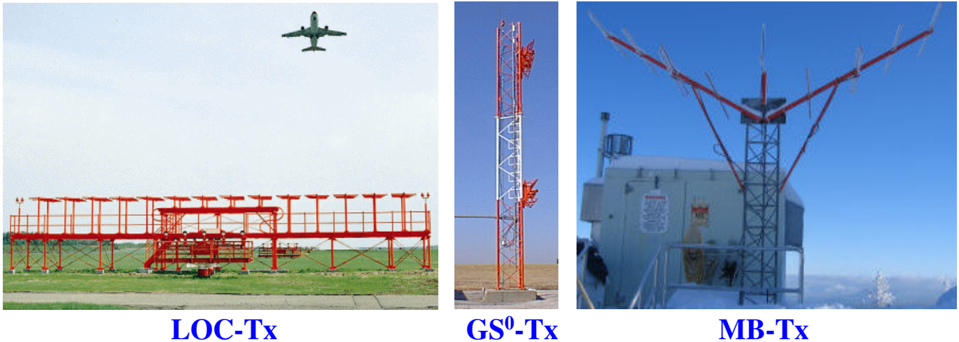
Figure-7.11 LOC, GS 0 , and MB-Txs [K5-5]
