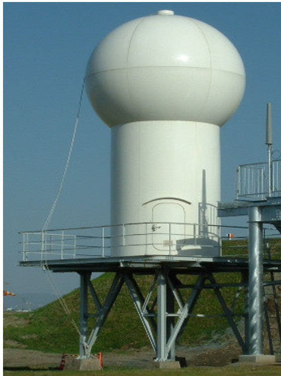
Figure-5.19 TACAN GND station [K4-7]
