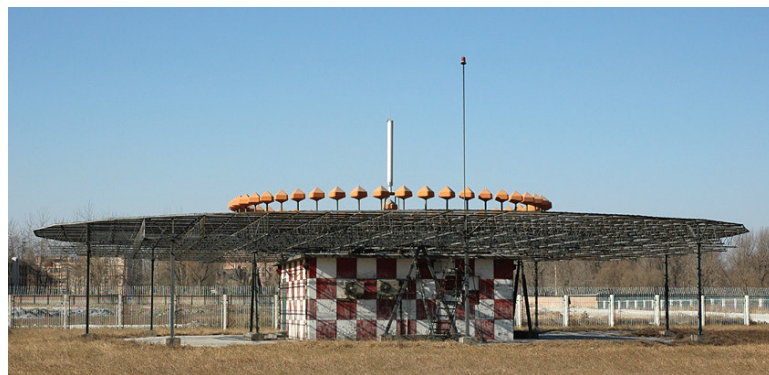
Figure-5.8 VOR GND station [K4-4]
